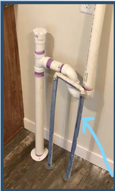
Water Softner Prep w/ Drain & Recept
